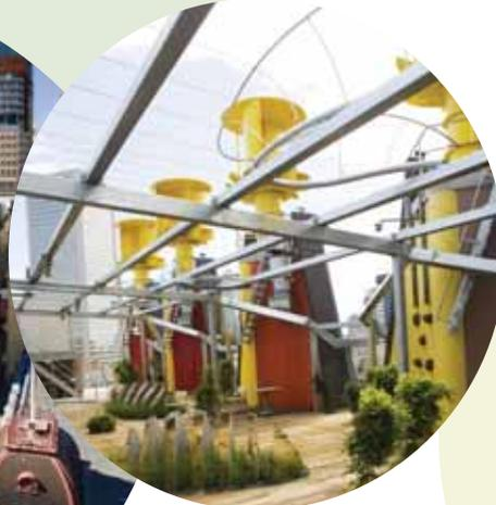
Melbourne City Council's CH2 building. Six wind-driven turbines atop the building assist with the exhaust air system and also generate power.
